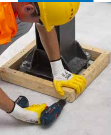
Assembling and mounting formwork before pouring mortar
